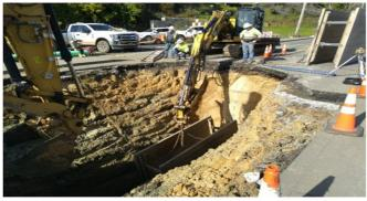
A portion of wastewater collection pipe failed this week, causing a  $12' \times 12' \times 5'$  deep void that had developed beneath the southbound lanes of Hwy 101. The depth of the pipe and the large void required both lanes of Hwy 101 to be closed which resulted in the need to reroute traffic.
